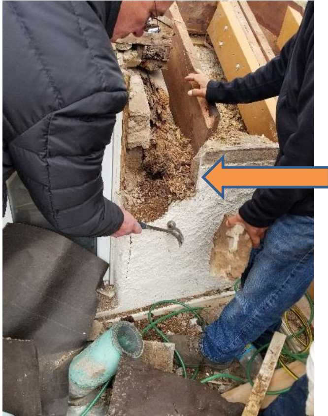
Note Deteriorated Masonry below Rafters
