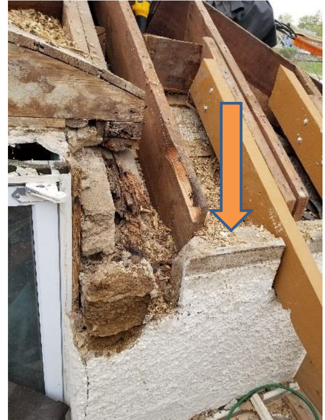
Note Section of Masonry Splaying Outward
