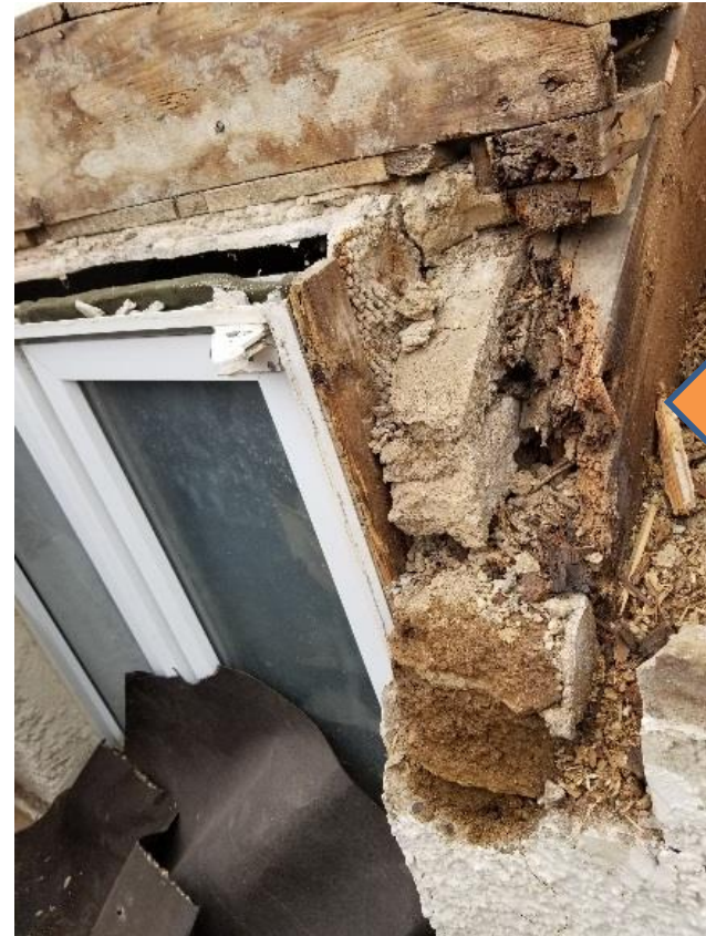
Note Deteriorated Double Rafter along Dormer Edge
