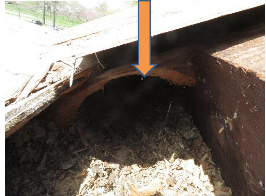
Note "Tunnel" Through Rafter
