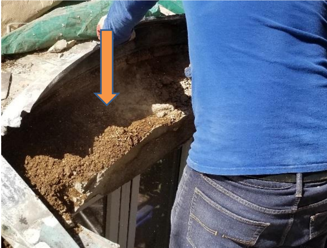
Note Disintegrating Cinder Block Backup
