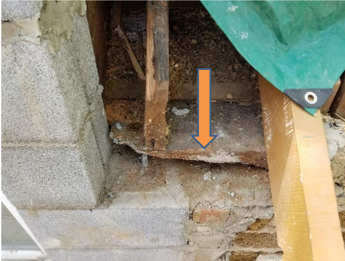
Note Deteriorated Sill Plate in Both Photos
